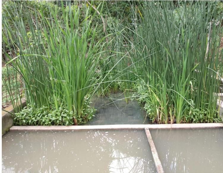
Figure 4. ERIS artificial wetland plant, single stage.
