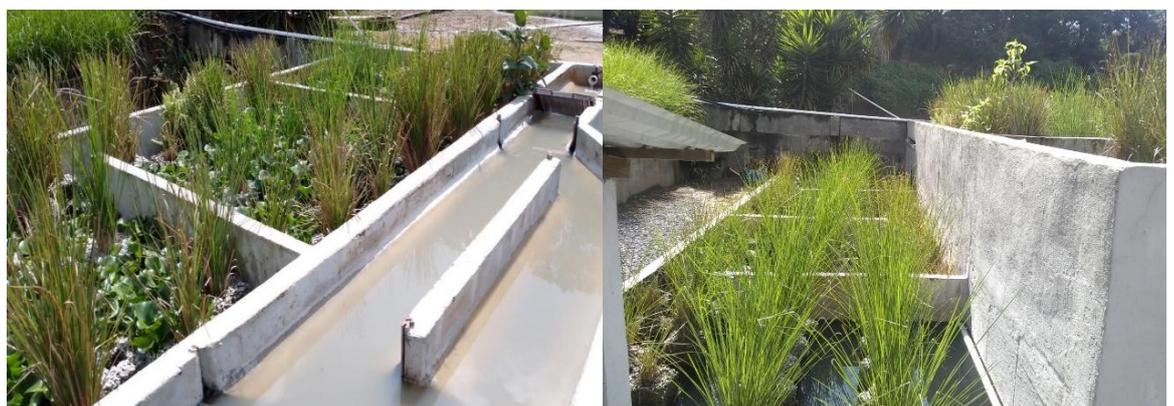
Figure 3. Artificial wetland plant belonging to the cement industry. Left stage 1, right stage 2.
